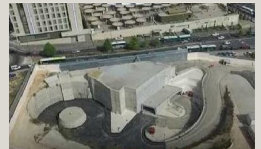
A view of what the new compound for the Israeli prime minister will look like when built. Photo: Channel 10.
