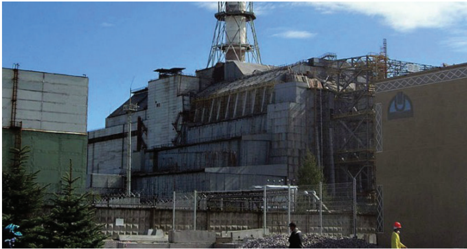
The Chernobyl reactor #4 building as of 2006, including the later-built sarcophagus and elements of the maximum-security perimeter. Photo: Carl Montgomery via Wikimedia Commons.
