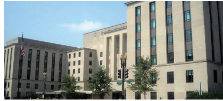
US State Department Truman Building. Photo: Wikimedia Commons.
