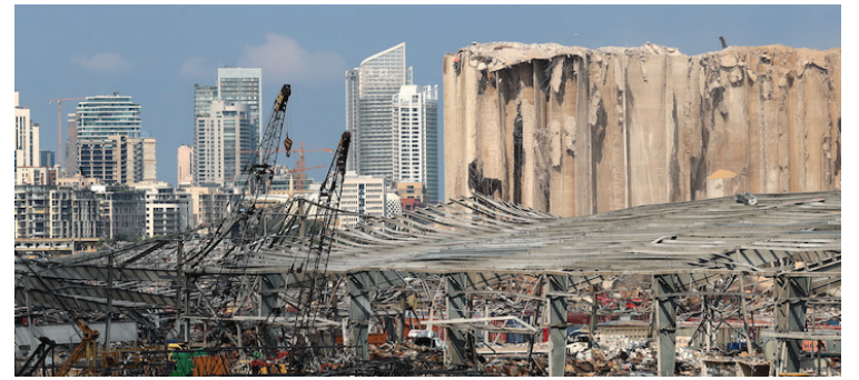
A view shows damage at the site of a massive explosion in Beirut's port area, Lebanon, Aug. 12, 2020. Photo: Reuters / Alkis Konstantinidis.
